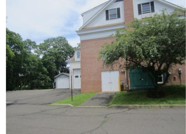
Cisterns can be installed at the southwest, west, and northeast corners of the building to capture and allow non-potable reuse of stormwater. Pervious pavement can be installed in the parking spaces southwest of the building to infiltrate parking lot runoff. A preliminary soil assessment suggests that more soil testing would be required before determining the soil's suitability for green infrastructure.
